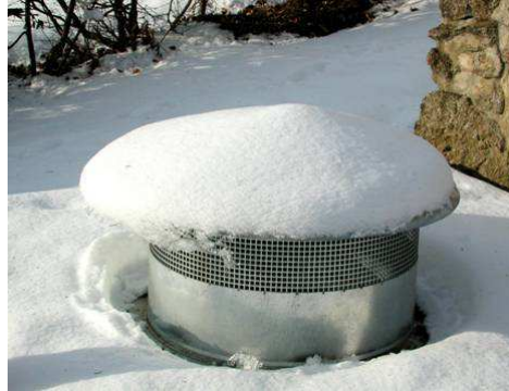
Ventilation system mit earth collector, heat recovery and fresh air preheating unit
