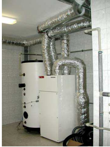
Ventilation system mit earth collector, heat recovery and fresh air preheating unit
