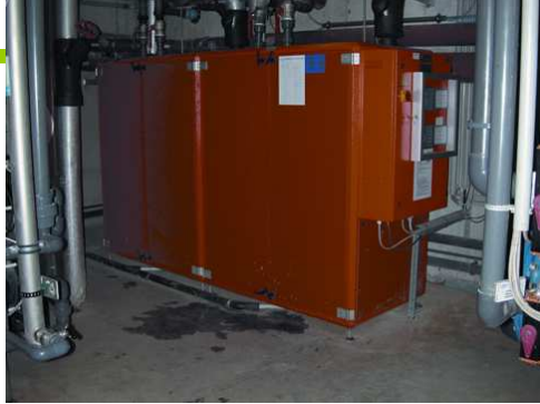
Menerga Heat Recovery from sewage Water with automatic Heat-exchange Cleaning
